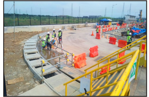
U-Ditch - Data Center, Cikarang
