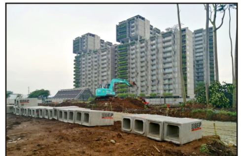
Box Culvert - Landmark Apartment, Bandung
