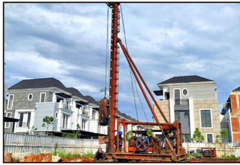
Pile - PT Graha Cipta Kharisma, Jakarta
