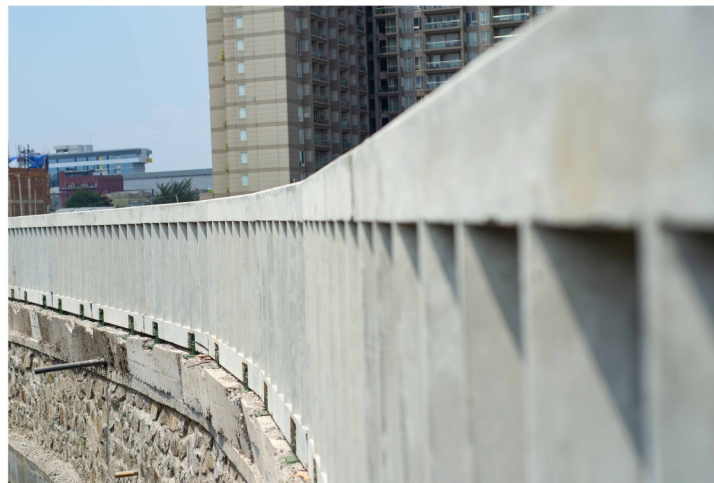
Precast Bridge Railing
